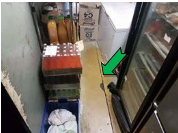
Photo 5. Interior, storage room, floor coverings – non asbestos-containing sheet vinyl.
