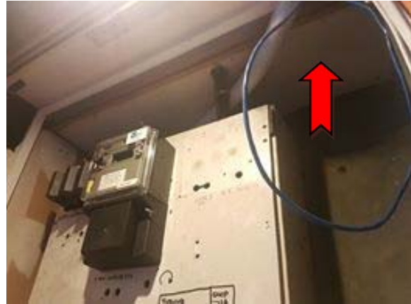
Photo 2. Interior, electrical distribution cupboard, lining – asbestos-containing fibre cement sheeting.
