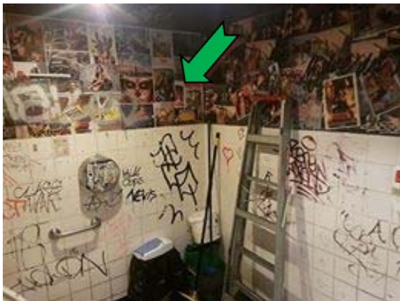
Photo 3. Interior, bathrooms, walls – non asbestos-containing fibre cement sheeting.
